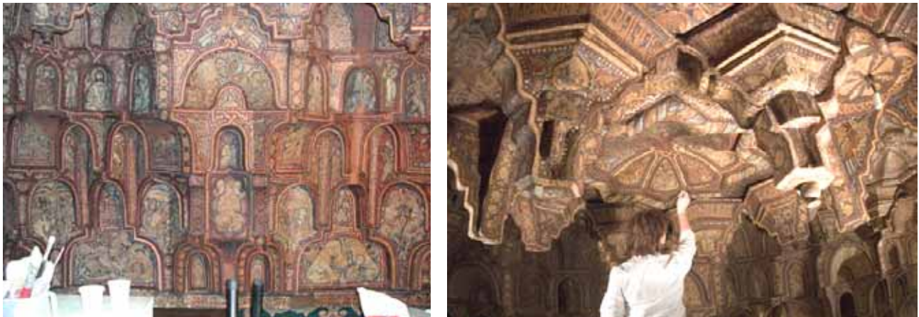
Fig. 3 – The muqarnas ceiling of nave: a particular of walls decoration and plane central portion, with its star-shaped and octagonal lacunars and stalactites.
