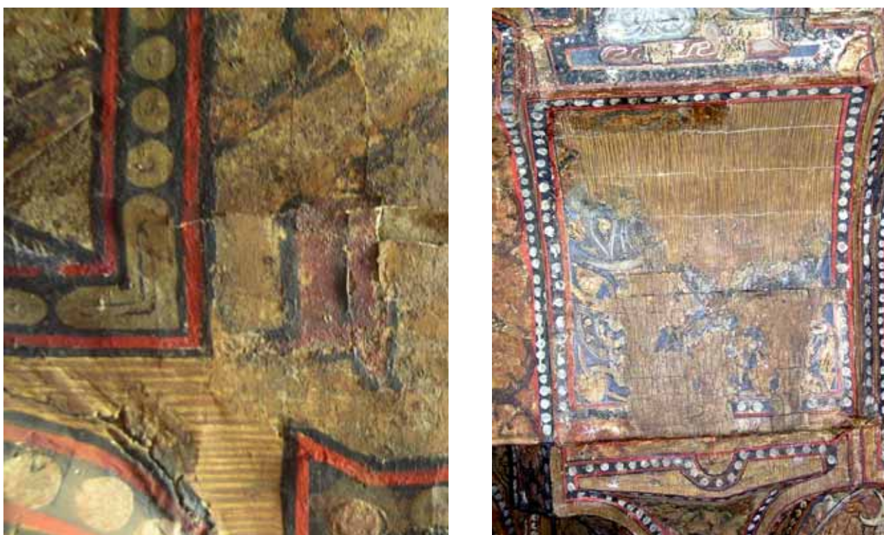
Fig. 7 – Liftings of preparatory layers and absence of the same preparatory layers e/o of colour, with integrations using the dash technique with chromatic decomposition ( rigatino ).
