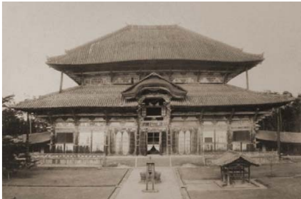
Fig.1 Main Hall of Todaiji Temple, condition before the repair works in 1891.
