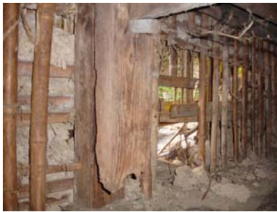
Figure 12. Exterior column base
