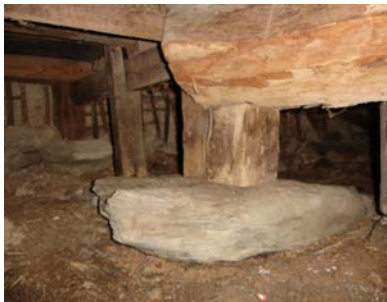
Figure 10. Foundation erosion
