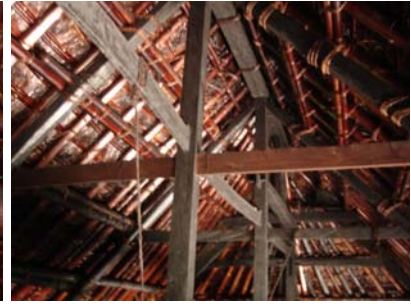
Figure 17. Warped braces
