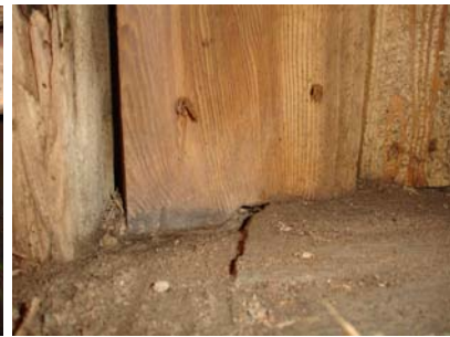
Figure 14. Column movement
