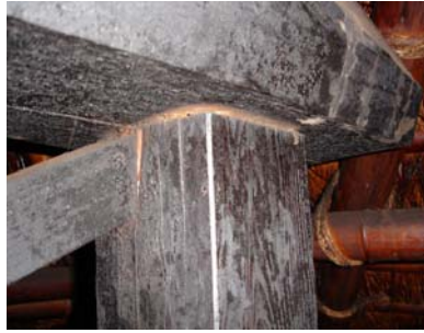
Figure 16. Stress cracks
