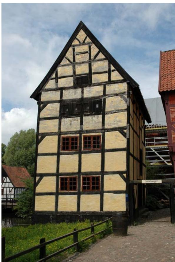
**Figure 4.** Detail of a house in Aarhus (Denmark): the floor beam on right is still in position in spite of its great deformation.
