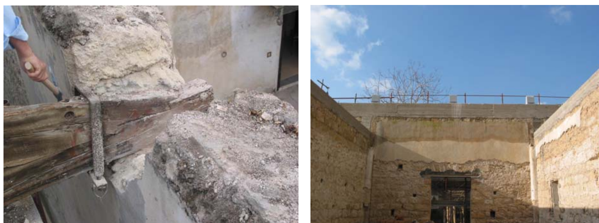
Figure 11. Dismantling of the head pieces from the masonry
