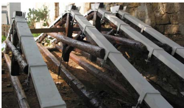
Figure 16. New metal structure connected to a pair of gusset plates
