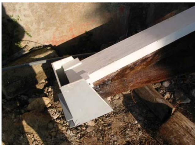
Figure 13. The steel shoe with the channel iron and the connection to the king post
