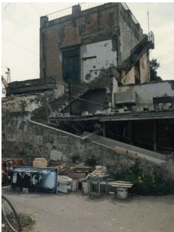
Figure 4. The north-west side of the building, that had crumbled
