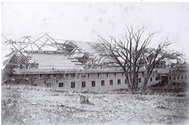
The main block of the building is approximately 32.6 meters wide by 127.4 meters long, with a two-story annex centered on the rear facade. The building is timber-framed, supported on foundation stonework of Monkton quartzite, and clad in wooden shingles.
