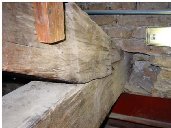
**Figure 4.** Joints details. Conjunction between the knee rafters and the tie beam. (N. Lombardini, 2007)
