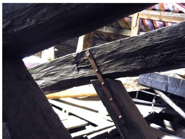
**Figures 6,7.** Examples of disjunctions between the struts and the knee rafter at several trusses (N. Lombardini, 2007)
