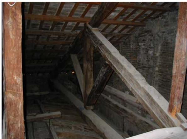
**Figure 2.** The trusses (N. Lombardini, 2007)
