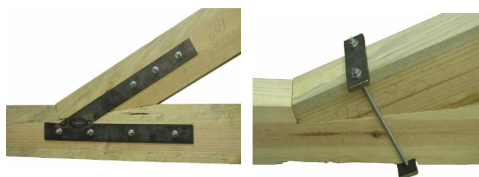
Figure 6. Stirrups and tension ties
