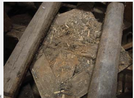
Figure 3 Skörstorp church. a) Rot damages. b) Some of the old repair measures. c) Wall plates were found to be more damaged than first assumed. d) Part of the beam system damaged by rot. Photo a, b and d: Carl Thelin. Photo c: author.
