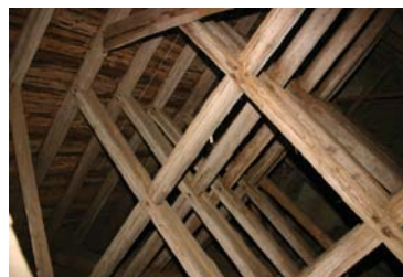
Figure 5 Marka church, roof trusses above the nave. Photo: Carl Thelin.
