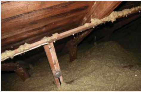
Figure 1 Threats to historic church roof trusses. a) Insidious, successive changes that transform the attic as a historic setting. b) Structural problems (the picture shows a material failure in a rafter). The dominating problem is the one where the trusses have lost their horizontal support. This leads to large stresses in rafters. c) Rot. d) Trusses are covered in insulation and become difficult to inspect.
